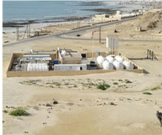
**Fig.2. Modern forward osmosis desalination plant at Al Khaluf, Oman.**
